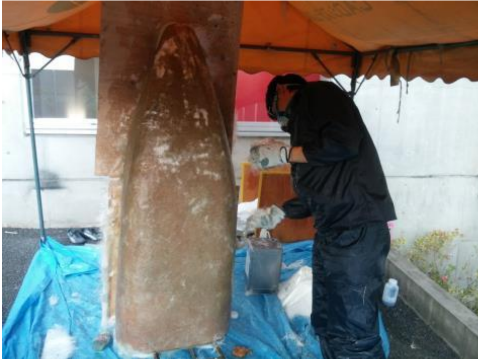
Fig1:GFRP 積層
